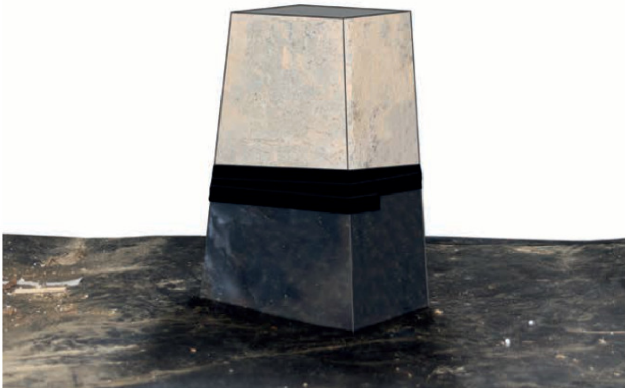
Figure 34 – On-ground vapour barrier folded up and taped around a pile
