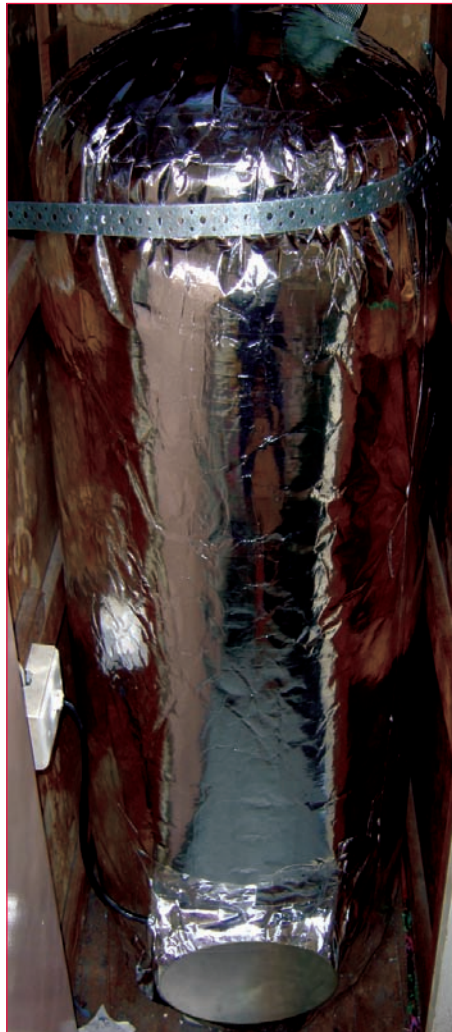
7 Completed installation with safety strap
